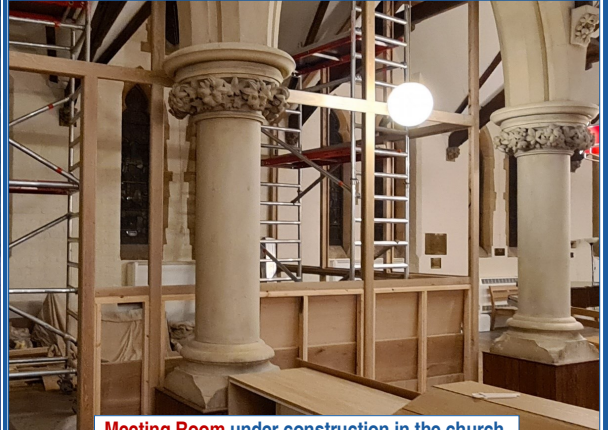
Meeting Room under construction in the church
