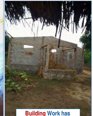
Building Work has begun on a new church
